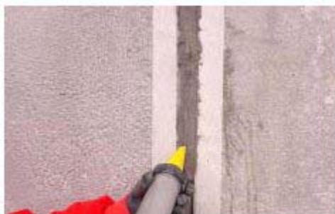
Application of MAXJOINT® ELASTIC
