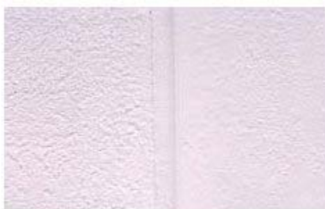
View of the finish joint. It can be painted with the desired colour.
