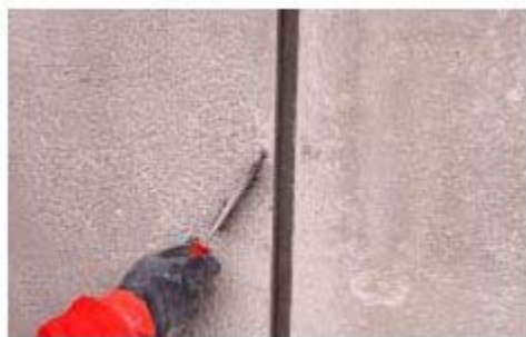
Preparation and cleaning of joint
